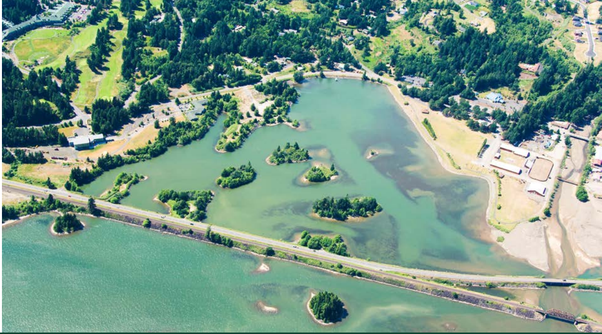
Figure 4.6-1 Rock Cove An aerial photo showing early sedimentation impacts from the Piper Road landslide Figure Credit: Department of Ecology (2007).
