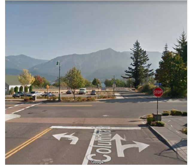
RE-ALIGNED COLUMBIA STREET
