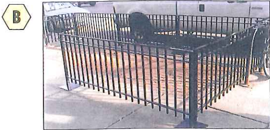
42" WLCC approved fencing
